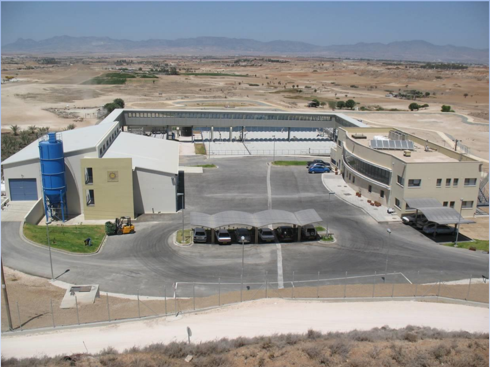
ANTHOUPOLIS WASTEWATER TREATMENT PLANT -SBN
