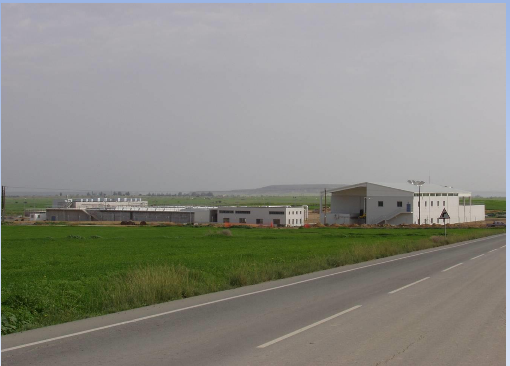
VATHIA GONIA WASTEWATER TREATMENT PLANT -SBN
